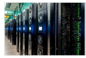
A row of racks with RDHxs connected to the same fluid loop as the CDU and PCL at <u>TACC</u>.
